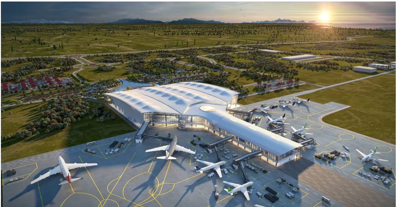
Bhogapuram International Airport (BIA) is a greenfield airport under construction in Visakhapatnam, Andhra Pradesh, India.
